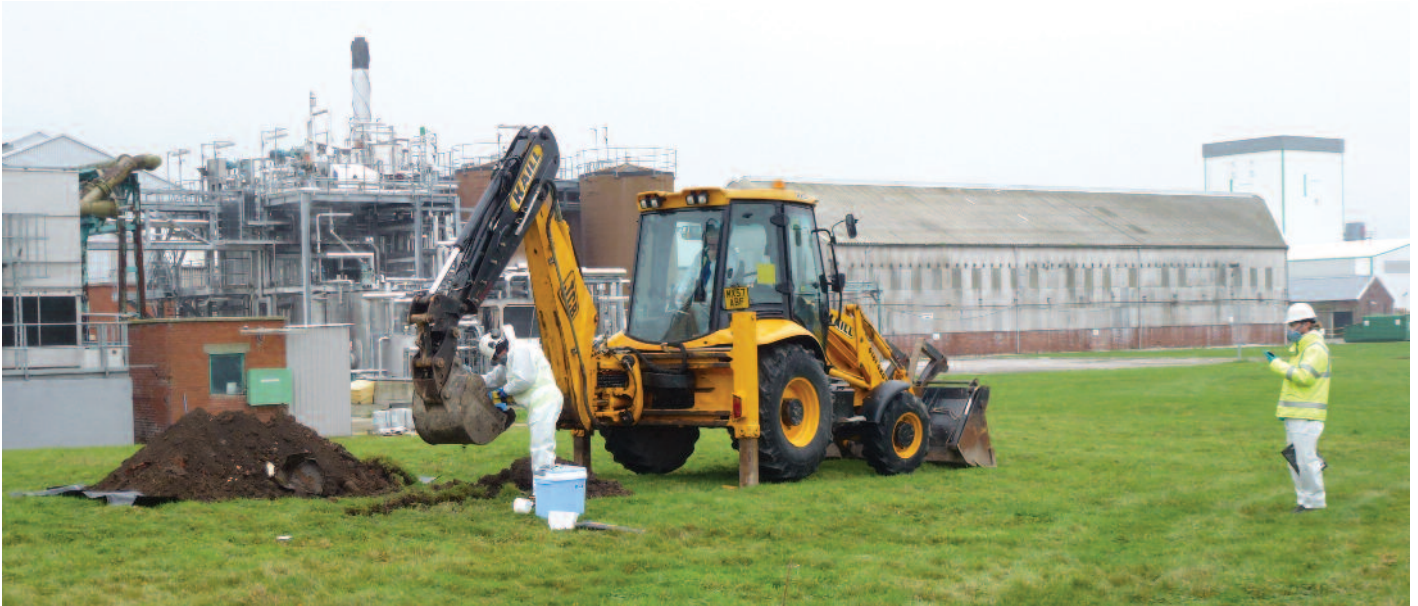
Ground investigation works underway at ThermPhos
