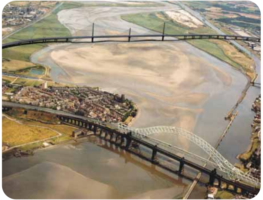
How the new bridge (top) will look next to the Silver Jubilee Bridge
