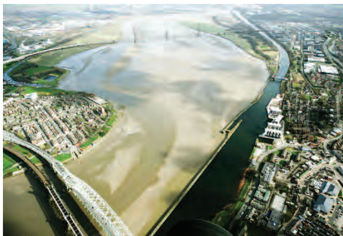
The new bridge alongside the Silver Jubilee Bridge
